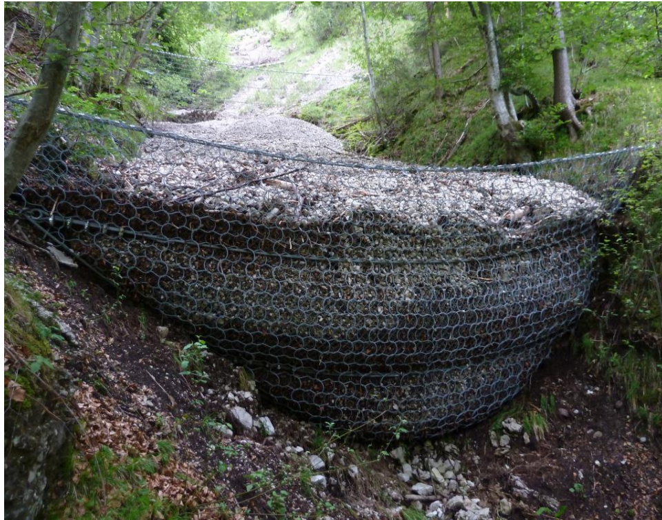
Depending on the nature of debris flow, varying mesh sizes can be used to filter out the desired fraction of debris. In this example, a fine mesh has been applied to the primary net structure to help retain the smaller particles.
