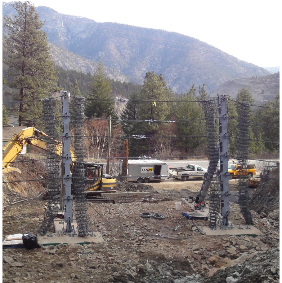
The Omega-Net packages allow for quick installation using no shackles to connect the bearing ropes. Once the bearing ropes are tensioned, the nets open like a curtain.
