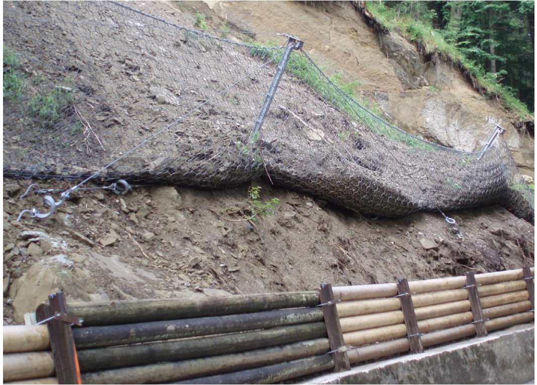
Shallow landslide barriers can be installed on steep slopes where stabilization methods would require more invasive techniques and often be too costly or unpractical.
