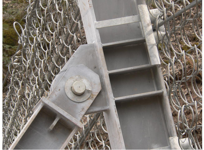
The hinge connection between the primary upright and the support brace, in this case made with a 70 mm pin.
