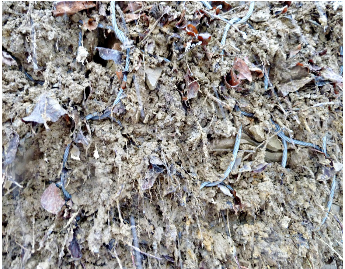
After the initial dynamic impact, material is retained by the cable nets and allowed to freely drain.
