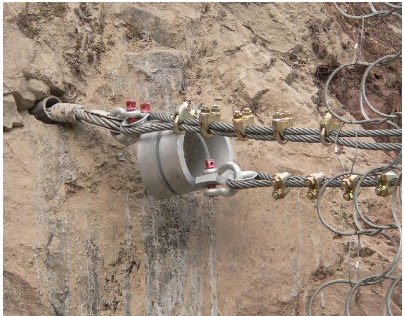
Wire rope anchors can be used to provide flexible anchorage. All connections are completed using high strength shackles and heavy-duty round thimbles for ease of installation and maintenance.
