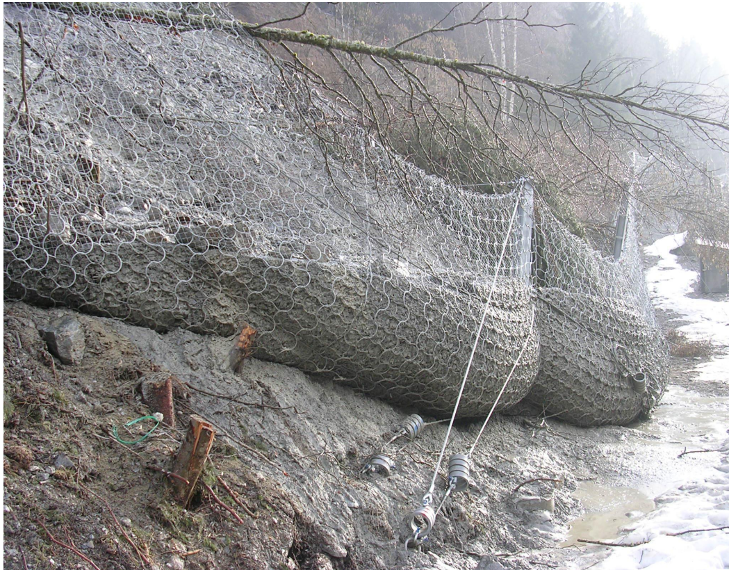
Following an event, the material can either be removed through access from behind the system or by opening the nets in the affected sections. It is not necessary to dismantle the entire system and most components can be re-used.
