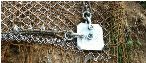
Corner plates are designed to receive bearing ropes using a shackle and thimble connection to ensure full strength and for ease of installation and maintenance.
