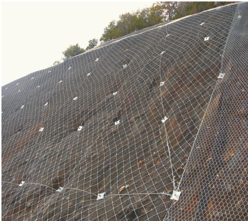
The Isofix system is used for both soil and rock slope stabilization.
