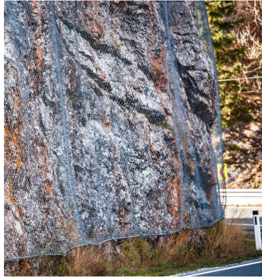
Draped mesh system using a rectangular netting that is supported only along the boundaries of the system.
