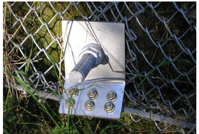
A non-positive/fixed connection to a boundary rope of a system.
