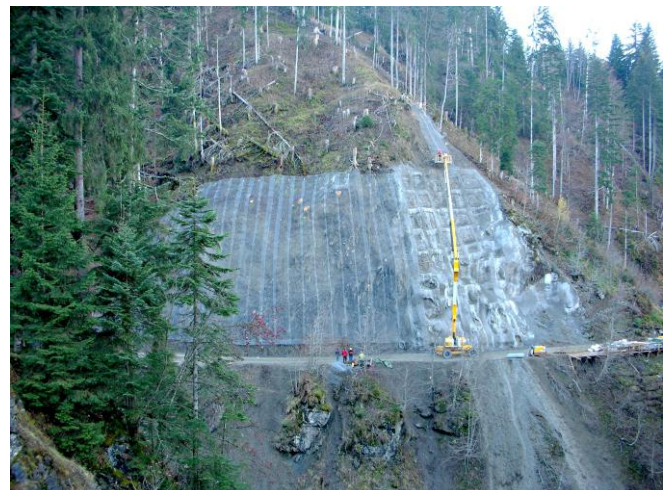
The light weight, long rolls make them ideal for covering large areas of slopes that are affected by unraveling and other mass wasting processes.
