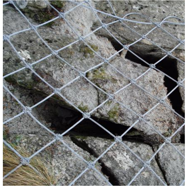
The unique Isostop clip provides a strong connection between crossing cables.
