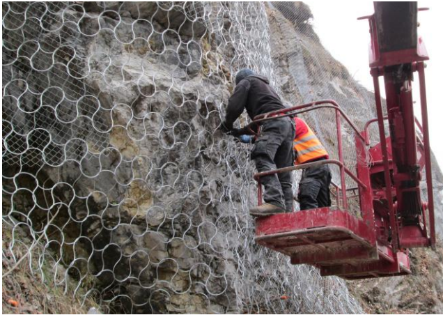
Installation of Omega-Net for slope stabilization.
