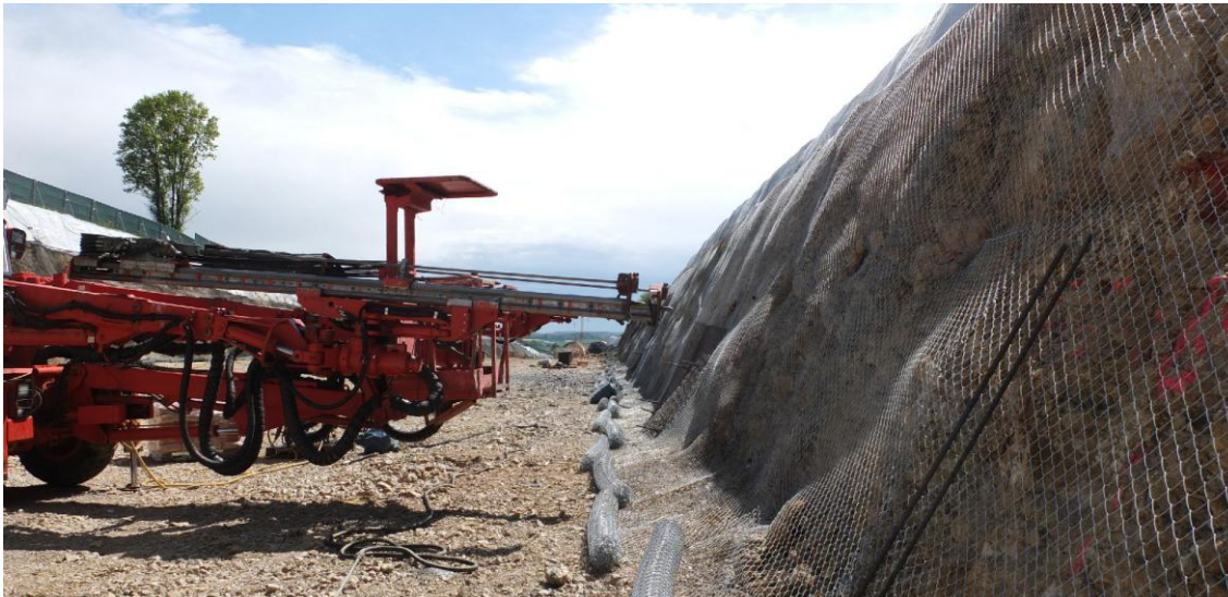
Slope stabilization using a combination of rectangular mesh and anchors.
