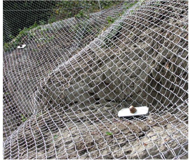
HPN+ is highly flexible which allows it to maximize slope surface contact.
