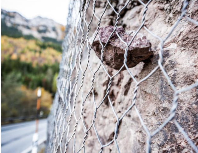
The thick, malleable wires used for hexagonal mesh, along with the twisted interlocking of the strands, yields a flexible product with redundancies.
