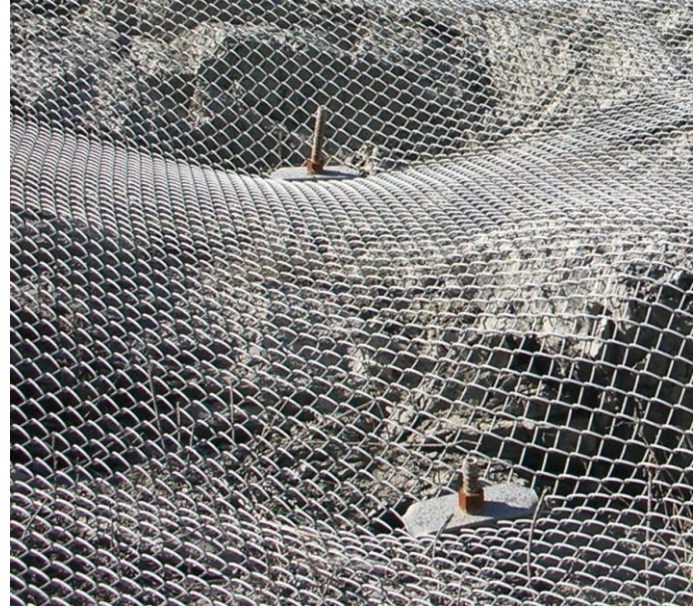
An example of interior anchors using a standard spike plate for the coupling. Anchor points are typically set in topographical lows whenever possible.
