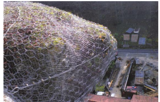
Heavy rock stabilization using Omega-Net.
