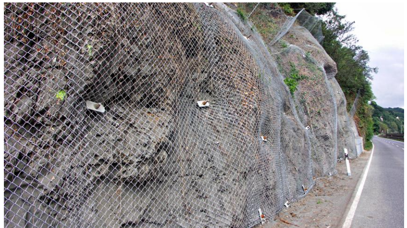
Slope stabilization works and low-energy rockfall fence using HPN+.
