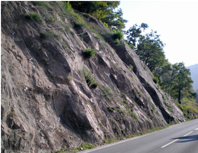
Hexagonal mesh can be used for slope retention systems where the forces are not high.
