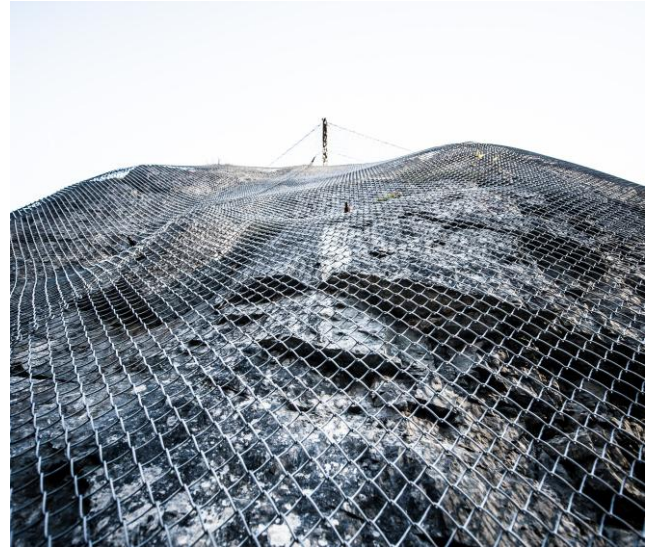
Rectangular netting lays flat against the slope and can conform to changes in topography better than hexagonal mesh.
