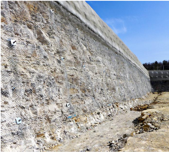
Rock wall reinforced using High Performance Netting.
