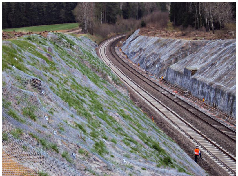
Railway cuts and existing walls stabilized using High Performance Netting.
