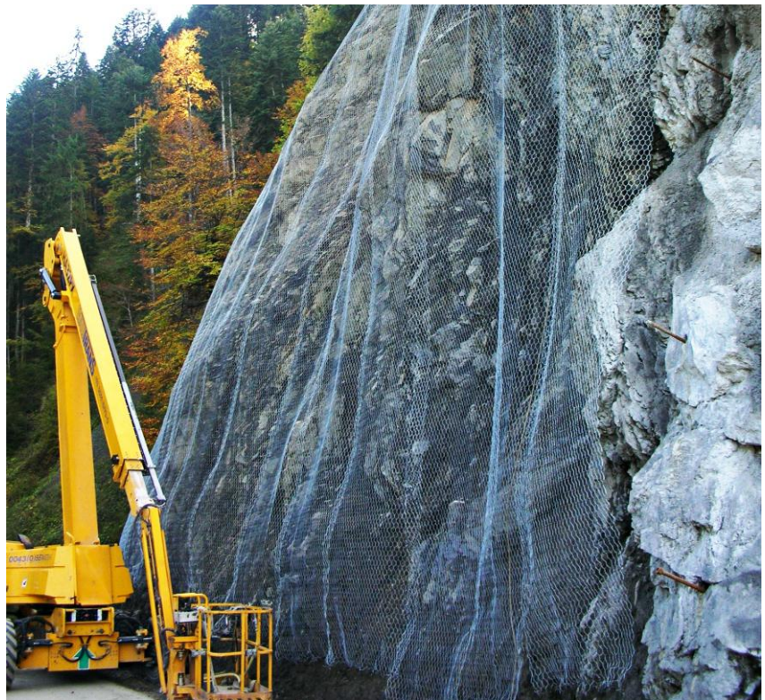
Example of a drape mesh system using hexagonal mesh.
