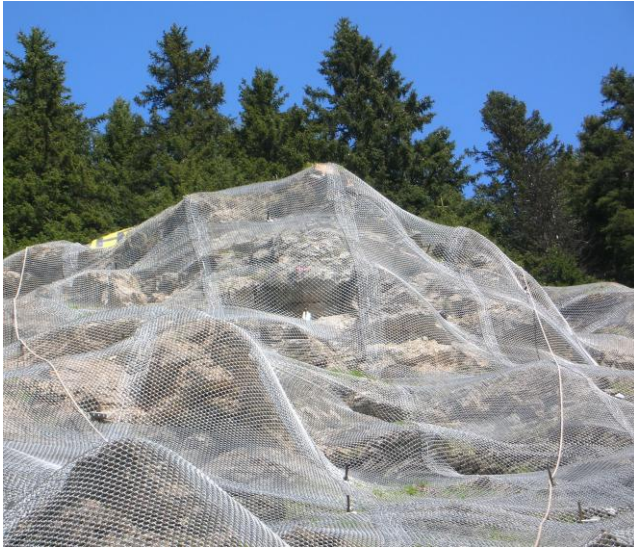
Due to its flexible nature, High Performance Netting can easily be fit to even the most challenging topography.
