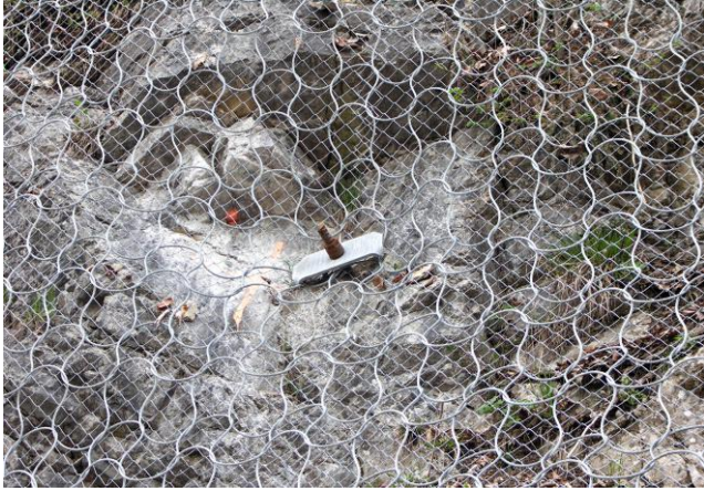
The Omega-Net can be made with a variety of mesh openings and wire diameters to best suit the strength requirements of the project.
